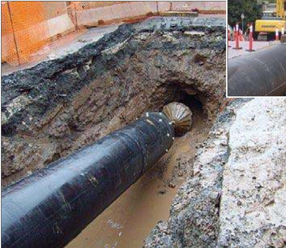
Right: Polyethylene pipe laid out before being hauled into the tunnel. Below: New 750mm diameter pipe enters the eye of the tunnel.
