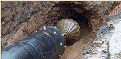
Drilling in Moncton . . . . . 8
