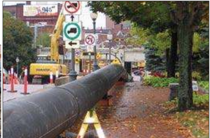
Right: Polyethylene pipe laid out before being hauled into the tunnel. Below: New 750mm diameter pipe enters the eye of the tunnel.
